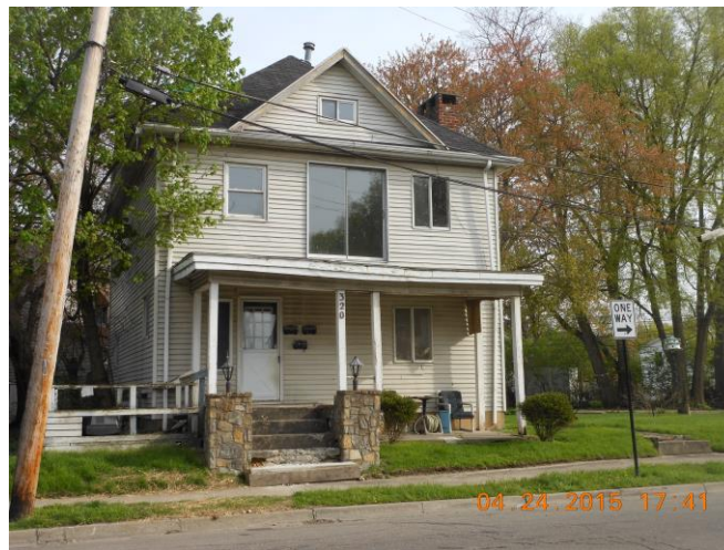
Subject Property: 320 N. Main Street – Front
